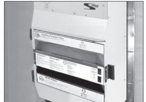
Figure 2.2b - Replace door and insert power cord into the receptacle of the HEPA and the other end into a wall outlet.
