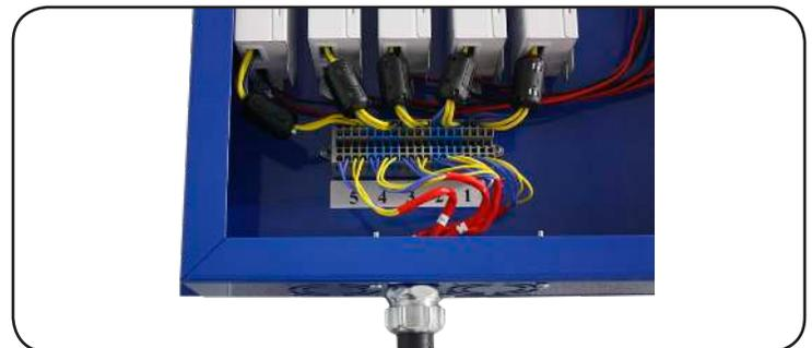
Refer to wiring diagram at the back of the cover of the ballast box. Using a small screw driver, press in the latch and insert the appropriate wire in the terminal block connector then release the screw driver. The wires should hold firmly into the terminal block connector.
